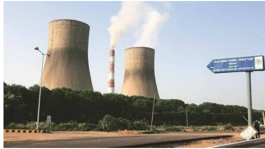
In October last year, India witnessed significant power shortages stemming from the low inventory of coal at the power plants. After seven months, we are back to square one as reports of coal-shortage induced power outages across states continue to pour in. On the one hand, there is a rush towards buying expensive coal and power on the exchanges. On the other, states like Andhra Pradesh and Gujarat have asked industries to reduce consumption to manage the power deficit. As economic activity resumed after the Covid-induced lockdowns, the
