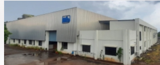
Menon Bearings Ltd. Plant Two MIDC, Gokul Shirgaon, Kolhapur. India
