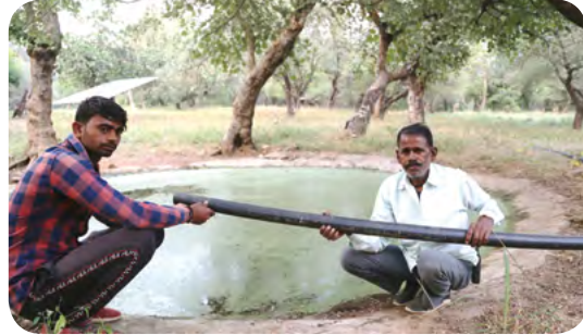
Solar pumps installation for providing water to wildlife at various places
