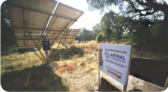
Pipeline project using solar powered water pumps to move rain water up so as to maintain water holes for the wildlife
