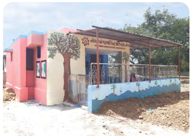
Renovation of old buildings of Angan wadi
