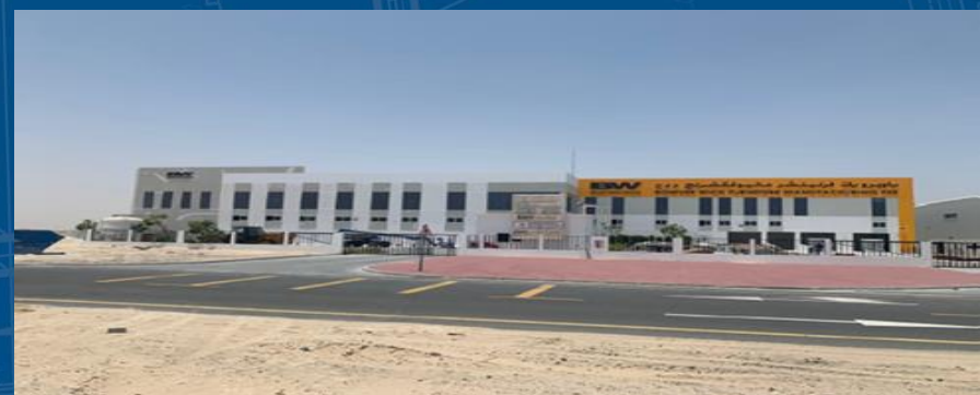
Bowyer Wick Office & Warehouse
