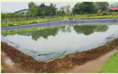
Construction of Multiple Farm Ponds Keshav Srushti Maharashtra
