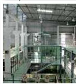
Polymer Manufacturing Unit, Patancheru, Telangana
