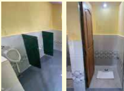
Construction of School Sanitation Unit Habitat for Humanity Maharashtra
