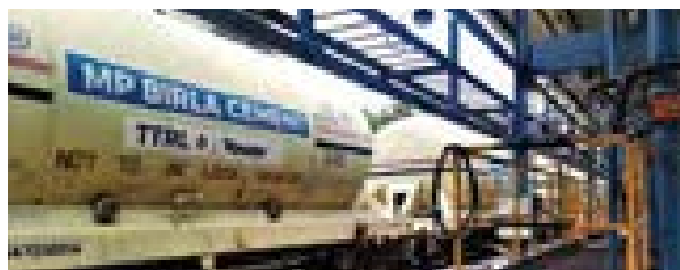
Maihar BTAP Wagon unloading facility
