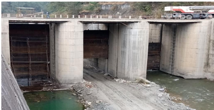
COMPLETE VIEW OF BARRAGE SERVICE, UNDER-SLUCICE GATE
