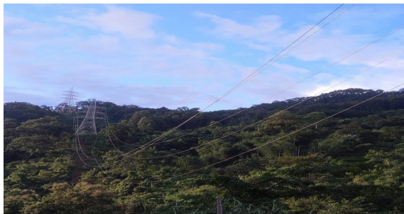
STRINGING WORK IN 220KV TRANSMISSION LINE 5.7KM COMPLETED
