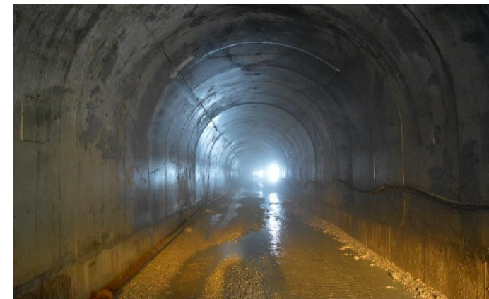
HEAD RACE TUNNEL COMPLETED
