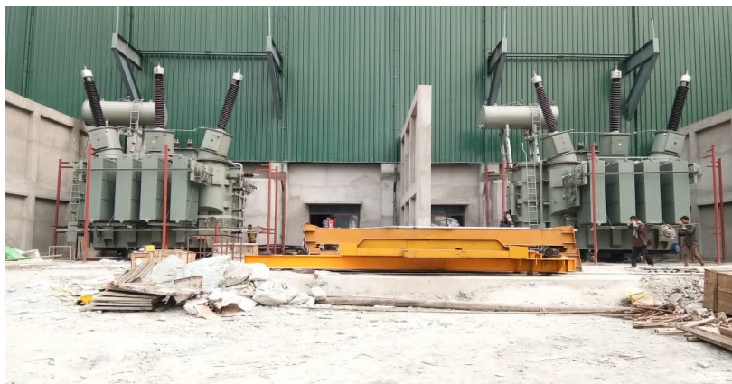
60/ 75 MVA GENERATOR TRANSFORMERS ERECTION COMPLETED
