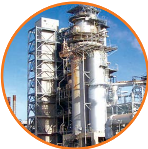
HPCL Bhatinda & Manglore Refinery Project Project-Refinery Project Products Used-Pipes
