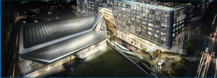
HVAC works in Doha Live, Qatar
