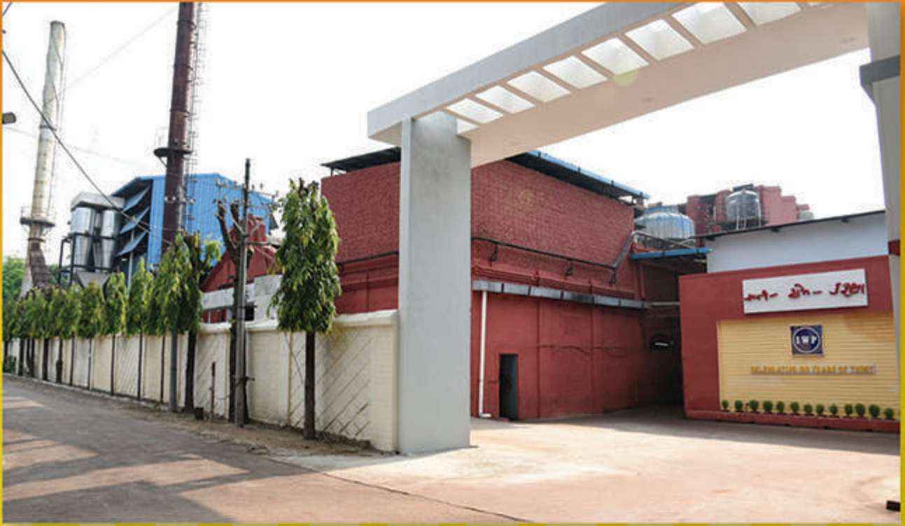
Plant at IZZATNAGAR, Barielly
