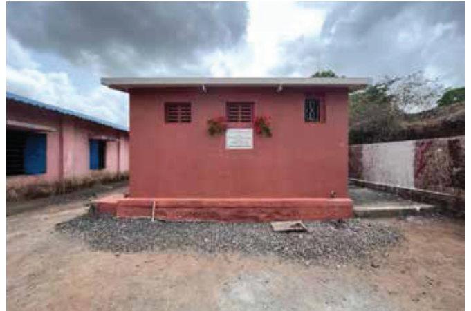
Construction of Toilet, Waalvihir School
