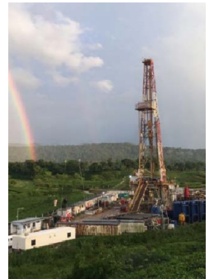
Ongoing Drilling Operations in Dirok Gas Field, Assam
