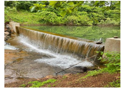
Completed water check dams, for water shed management in drought prone areas near Nashik
