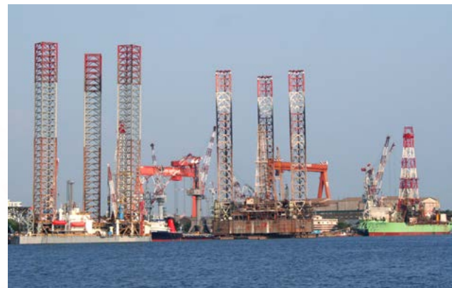
Oil Rig Upgrades, Repair Projects, and Conversions
