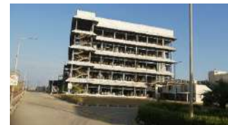
Specialty Fluorochemicals facility (Dahej, India)
