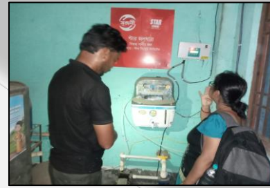
Water System Checking
