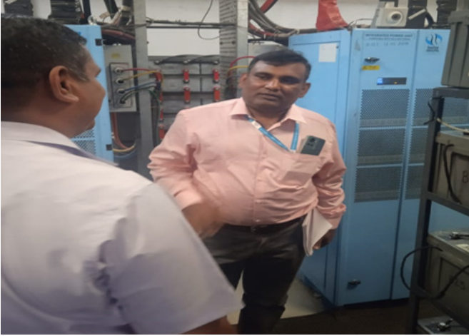
Inspection at Mahalaxmi PoP, Mumbai
