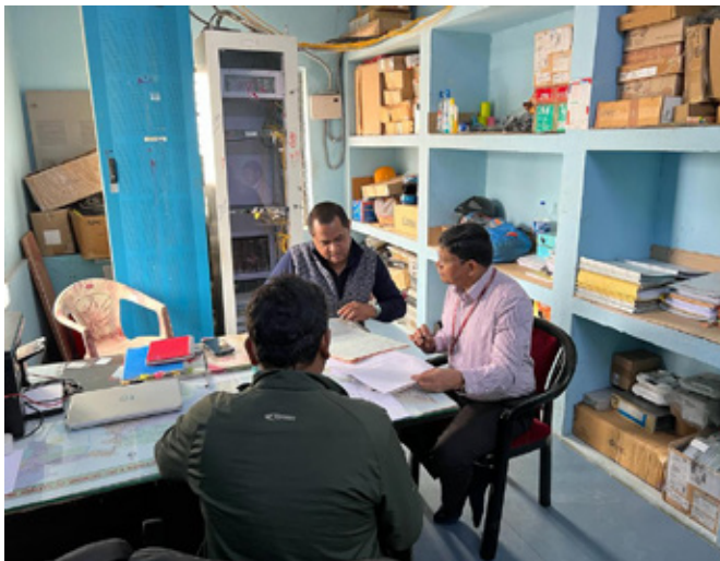
Inspection at Cuttack PoP
