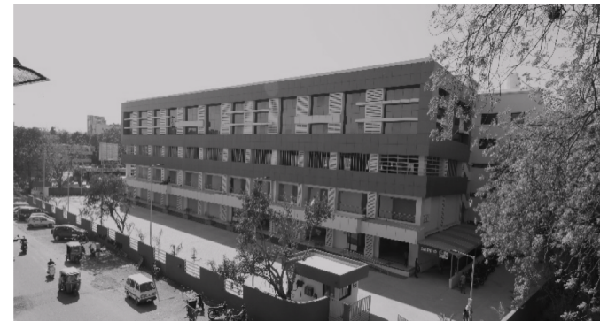
Multi-storied parking at Navrangpura, Ahmedabad
