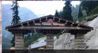
Atal Tunnel, India
