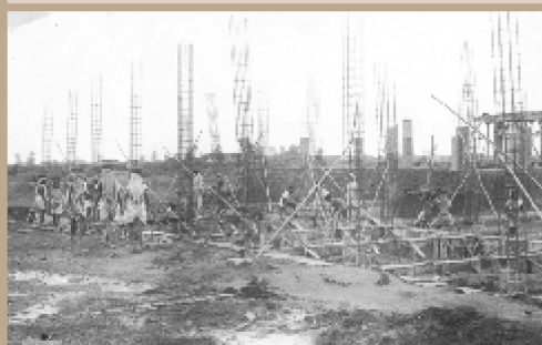
FACTORY BUILDING CONSTRUCTION
