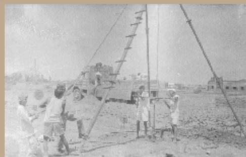
PILING-BEGINNING OF CIVIL CONSTRUCTION
