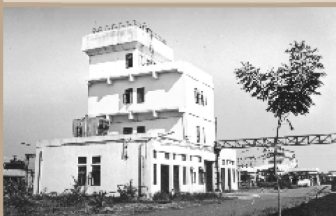
CHEMICAL PLANT - TUNGSTEN ORE TO APT
