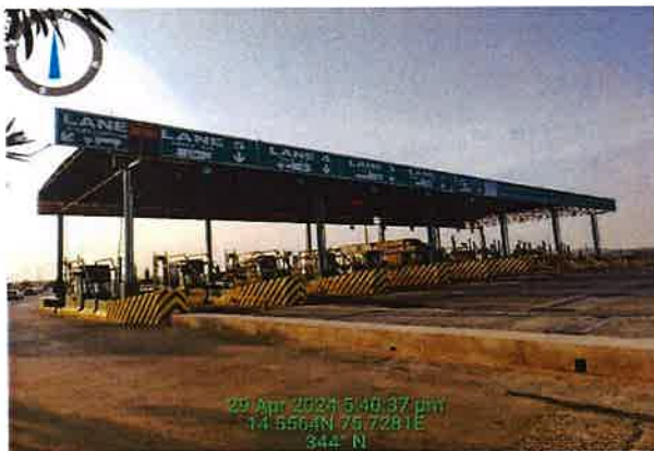
Chalageri Toll Plaza
