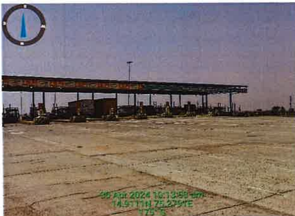
Bankapur Toll Plaza
