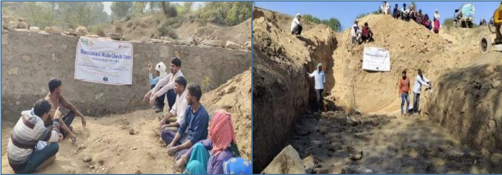
Check dams being constructed in Alwar district to catch and channelize rain water. Another sustainable initiative is to channelize and save water through a project of "Water conservation through installation of rainwater harvesting structures in the form of check dams and gabion structures" in Alwar, Rajasthan. PFS has funded four check dams and two gabion structures to improve ground water situation in the area.
