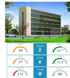
INDOOR AIR QUALITY DASHBOARDS ACROSS ASSETS
