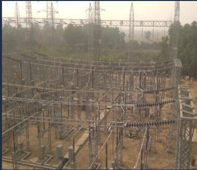
DVC Parulia, West Bengal- Commissioning of 220kV AIS Line Bays
