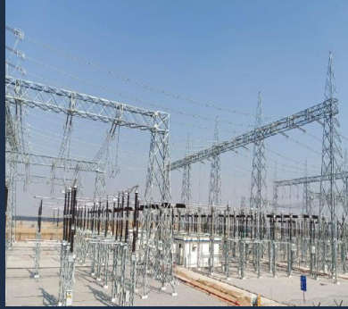
Avaada(Bikaner), Rajasthan- Commissioning of 150 MVA transformers & 400kV AIS bays
