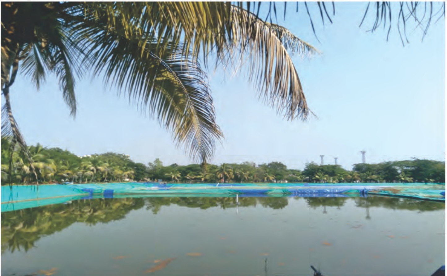
Glimpse of our Rainwater harvesting pond at Gadegaon, Maharashtra
