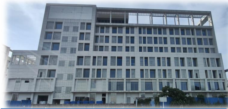
Taj Cochin Airport (Under Construction)
