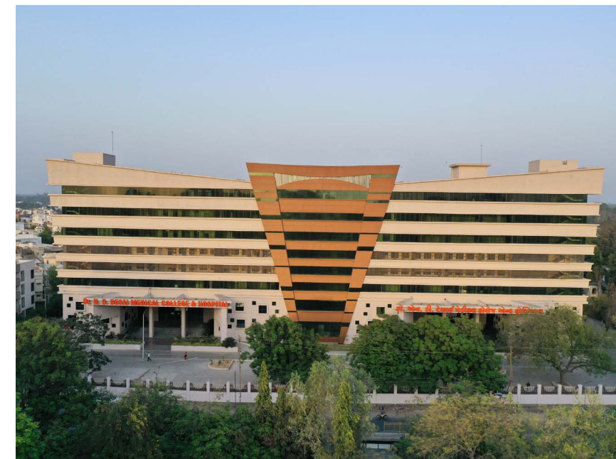
Super specialty hospital located at Nadiad, Gujarat
