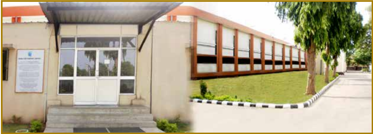
Kanjari Factory - Gujarat
