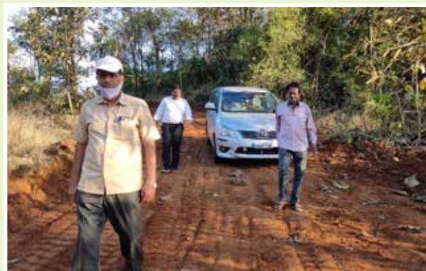
Road Construction, Vadad, Guhagar, Ratnagiri
