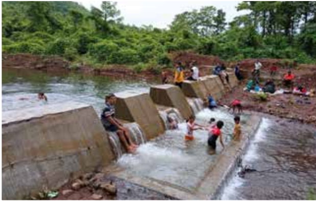
Water Project - Impact: Talaghar, Roha, Raigad
