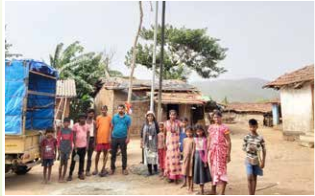
Solar Street Light - Garbat Adiwasi Wadi, Roha, Raigad
