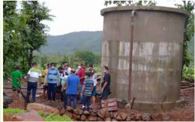
Drinking Water Facility: Sakhar, Khed, Ratnagiri
