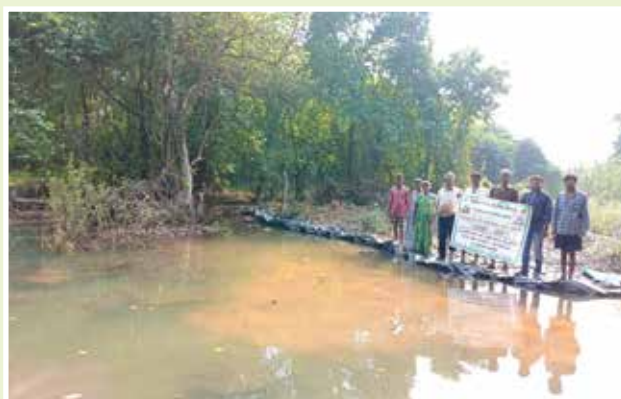
Check Dam:Moravane, Chiplun, Ratnagiri
