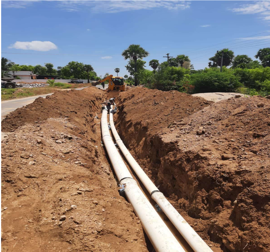
LIFT IRRIGATION PROJECT, BELGAUM
