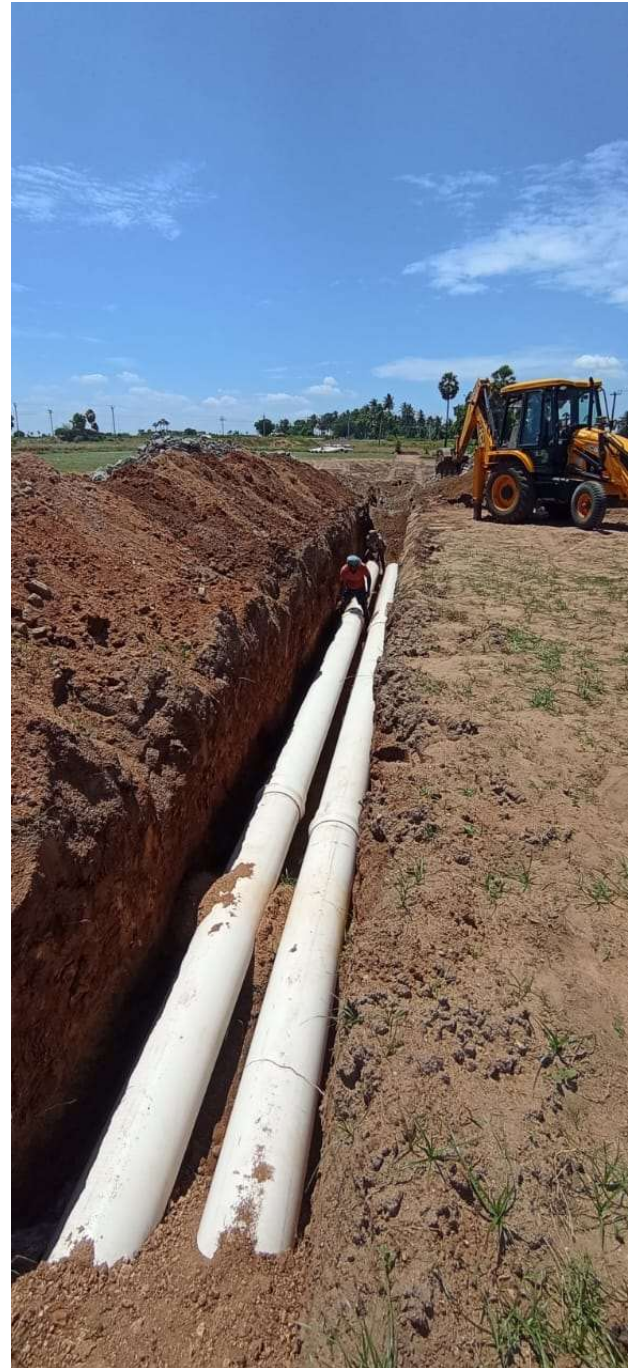
LIFT IRRIGATION PROJECT, ERODE
