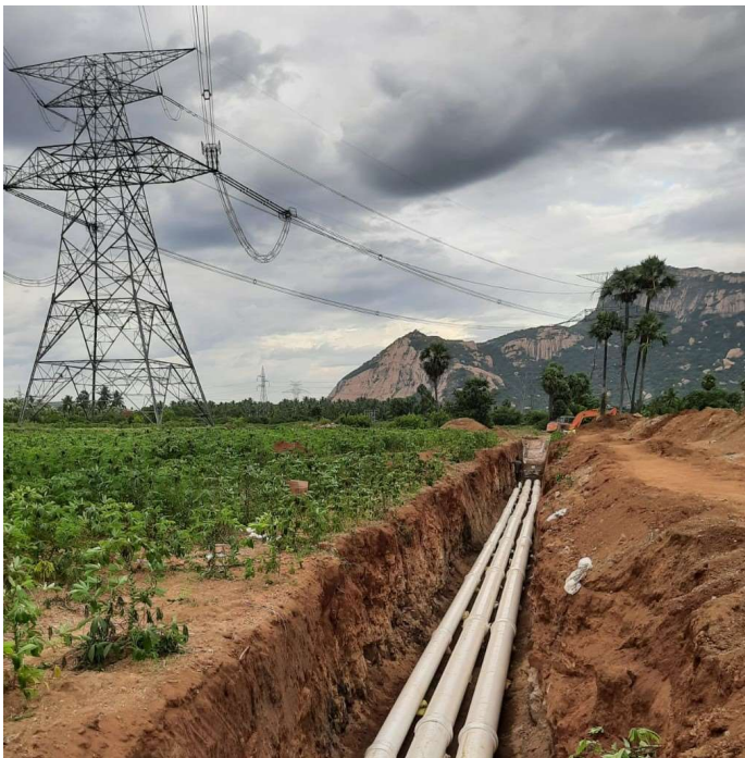
LIFT IRRIGATION PROJECT, TIRUCHENGODE
