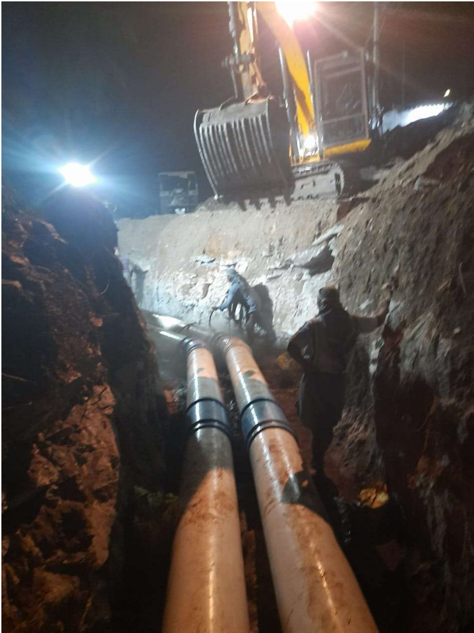
LIFT IRRIGATION PROJECT, COIMBATORE
