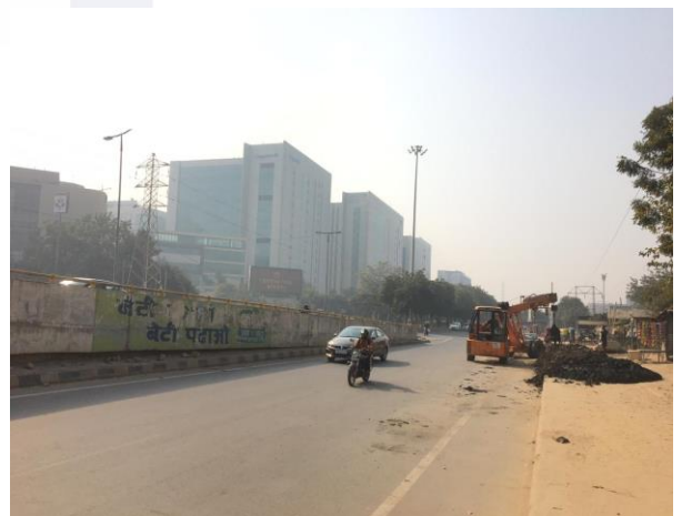
View of the Access Road
