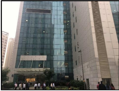
View of Tower 6
