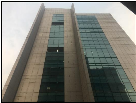
View of Tower 4
