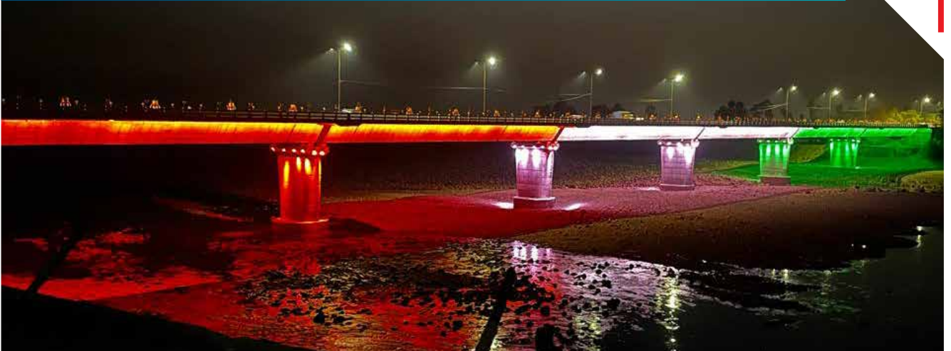
TAWI RIVER BRIDGE, JAMMU
