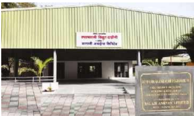
Set-up of ME- Electrical Cremation Furnace of cost of ₹1.05 Crore on 26.01.2022
