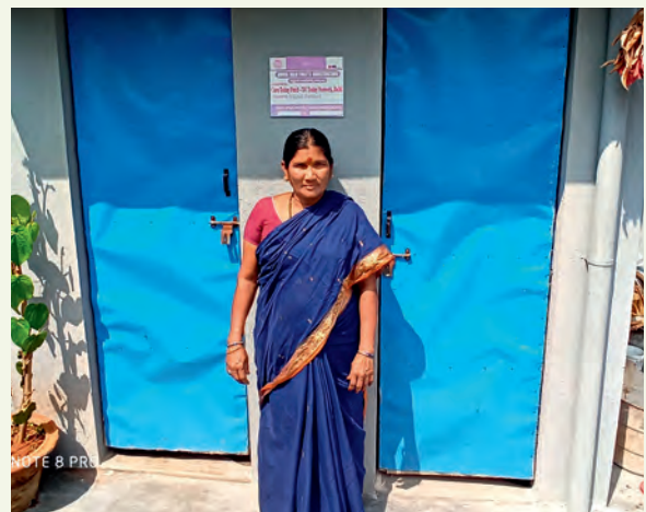
Ms. Achiyamma Kothalanka from village Thotada in Vishakapatnam district, Andhra Pradesh in front of her newly constructed household toilet and bathroom.
