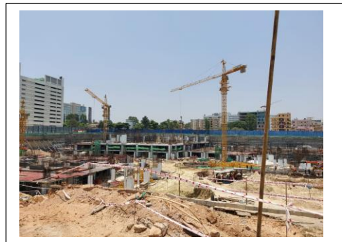
View of under construction Block 8 at the SP
