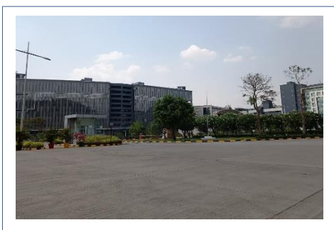
View of front façade for Under Construction Blocks ~ Hudson & Ganges
