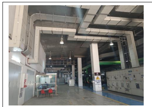
Internal view of Maintenance area, work in progress – Epoxy flooring
