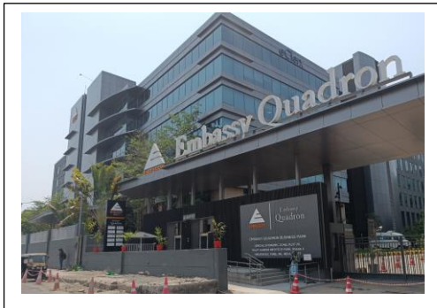
External view of the subject property (SP) ~ Entry Gate and Block 1
