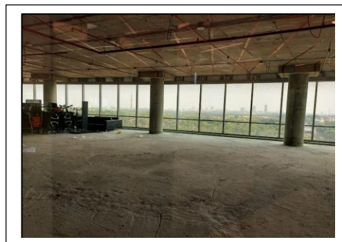
Internal View of office area
