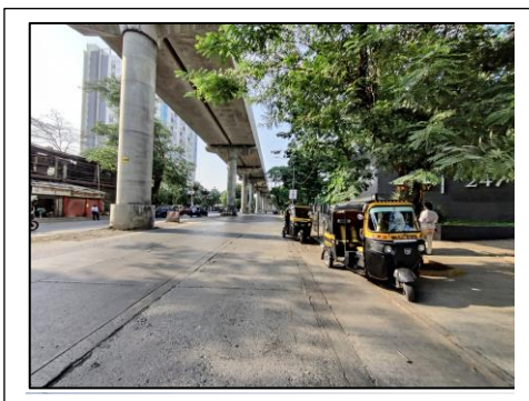
View of the primary access road/entrance
