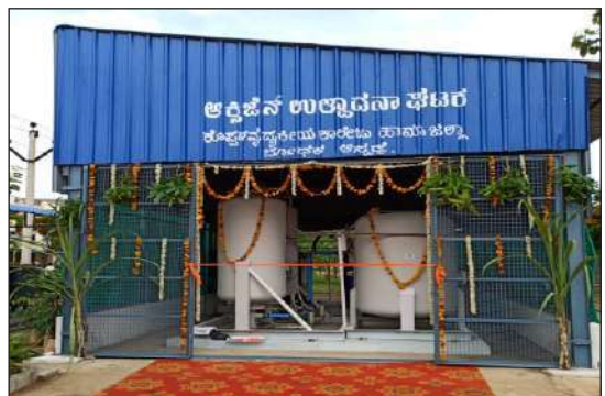
Medical Oxygen Plant
