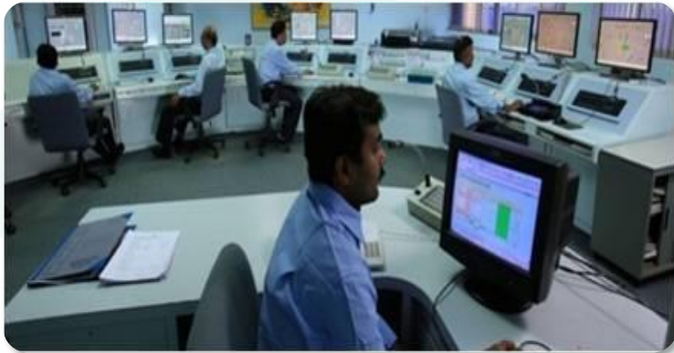
Control Room - Taloja
