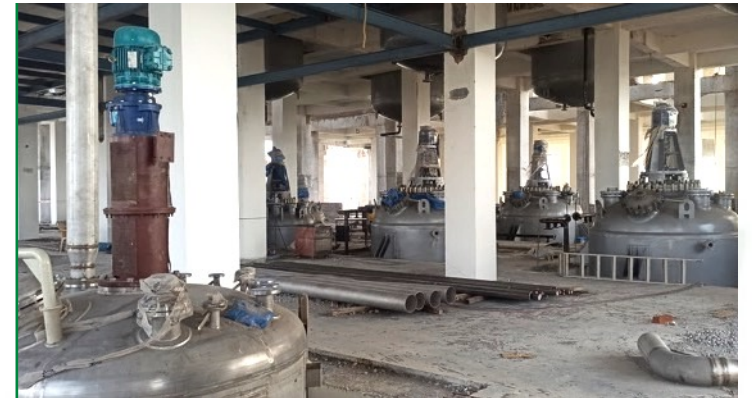
Reactors Installed & Piping Commenced
