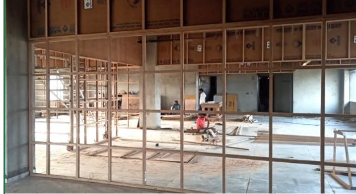
Furniture Work at R&D Laboratory and Administration Office
