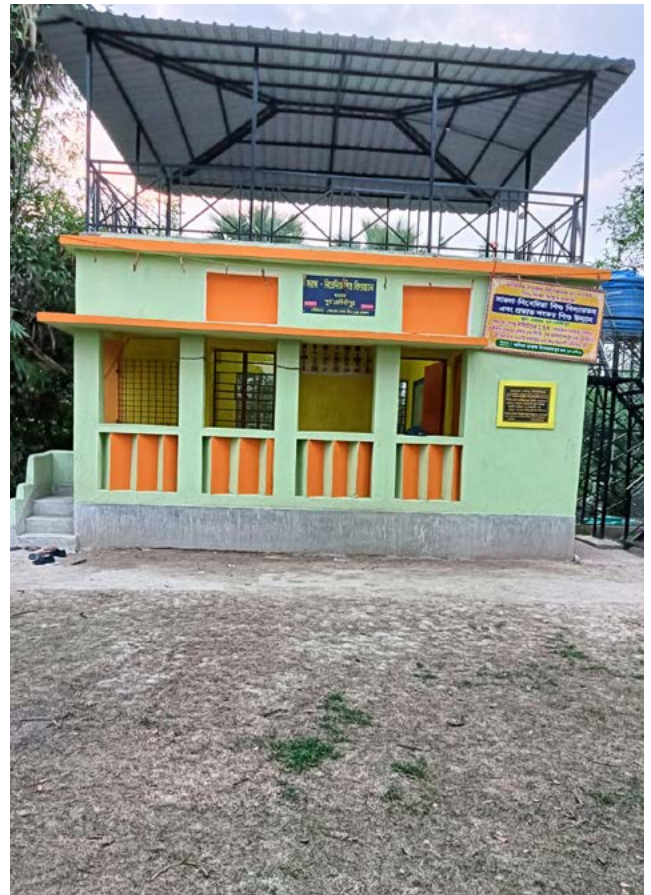
Reconstructed Creche-cum Pre-primary Education Centre at Mayachar Village
