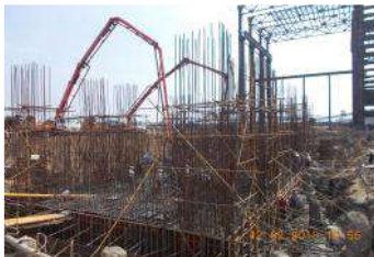
1X800 MW TPSS , CIVIL, STRUCTURAL WORKS, NORTH CHENNAI, BHEL
