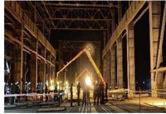
1X800 MW TPSS, CIVIL, STRUCTURAL AND ARCHITECTURAL WORK STAGE-3, NORTH CHENNAI, BHEL
