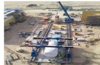
1519 MW FADHILI CCPP, SAUDI ARABIA GTG,STG & BOP INSTALLATION
