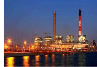
BOILER, ESP, TG AUXILIARIES, UMPP 800 MW, GUJARAT, TATA POWER (COMPLETED)
