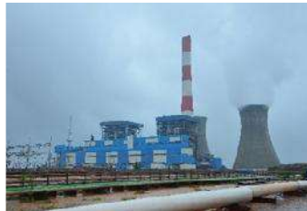
2X600MW TPP, BOILER & STG, MANGALORE, LANCO (COMPLETED)
