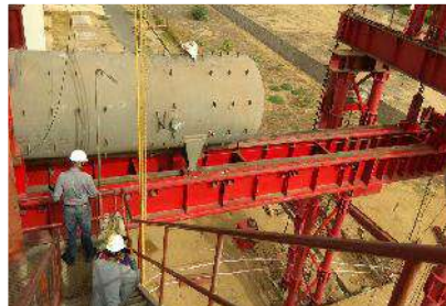
HP HEATER REPLACEMENT 800MW ,CGPL MUNDRA2
