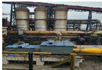
BLAST FURNACE, STEEL PLANT WORK, JSPL, ANGUL
