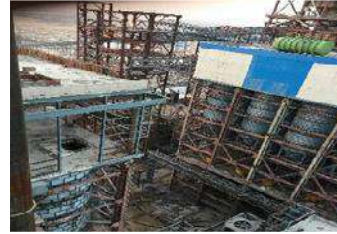
2X660 MW TP9, CIVIL, STRUCTURAL & ARCHITECTURAL WORK UNIT-7 & 8, SURTGARH, BHEL
