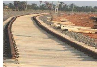
GDV-MTM 37 ,DOUBLING & ELECTRIFICATION WORKS , RVNL
