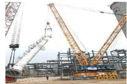
UREA REACTOR TANK INSTALLATION AT RAMAGAUNDAM, TELANGANA
