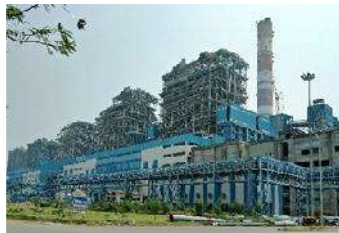
3X660 MW STPP, BOILER & CRITICAL PIPING, U#1,2&3, BARH, DOOSAN
