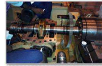
228MW, STEAMTURBINE,SABIYA, KUWAIT, MAIN OIL PUMP OVERHAULING
