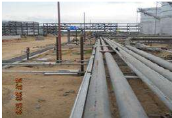
3X366 MW CCPP, CIVIL, STRUCT. & ARCH. WORK, IOCL PARADIP, BHEL
