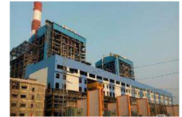
2X800 MW, YTPS, CIVIL, STRUCTURAL AND ARCHITECTURAL WORKS RAICHUR, BHEL (COMPLETED)
