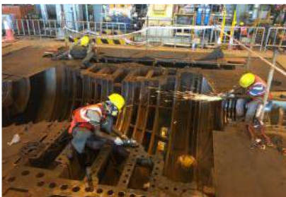
MAIN TURBINE OVERHAULING ,660 MW KAWAI
