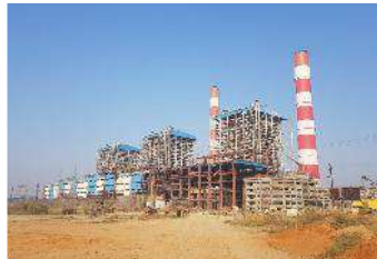
3X660 MW ,BOILER, ESP,CP, STRUCTURE & STG, NABINAGAR, BHEL
