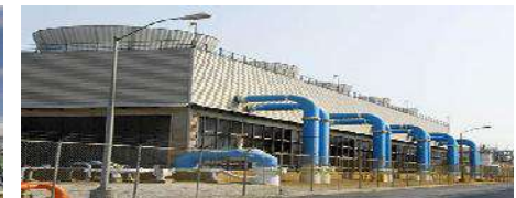
Infrastructure Construction (Civil)
