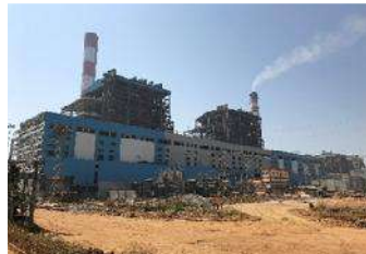
2X660 MW IBTPS, STRUCTURE & STG, BANHARPALLI, BHEL
