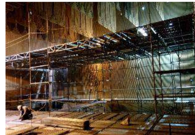
CUPLOCK SCAFFOLDING ERECTION 800MW,MUNDRA
