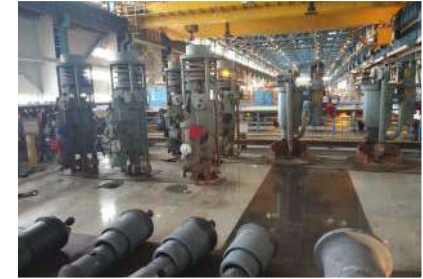
CONTROL & STOP VALVES OVERHAULING SIPAT 660MW
