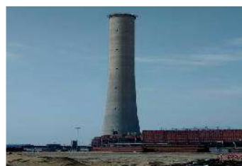
1X500 MW, FGUTTP, CIVIL, STRUCTURAL AND BOP & CHP, UNCHAHAR, NBPPL
