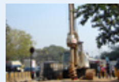
Hydraulic piling rig
