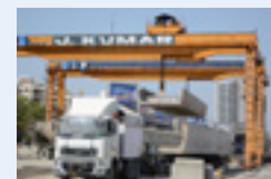
Casting yard (Elevated metro)
