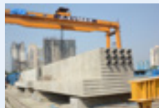
Casting yard (Underground metro)
