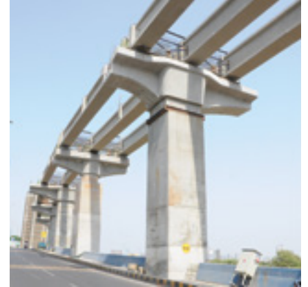
Mumbai Metro Line 2B
