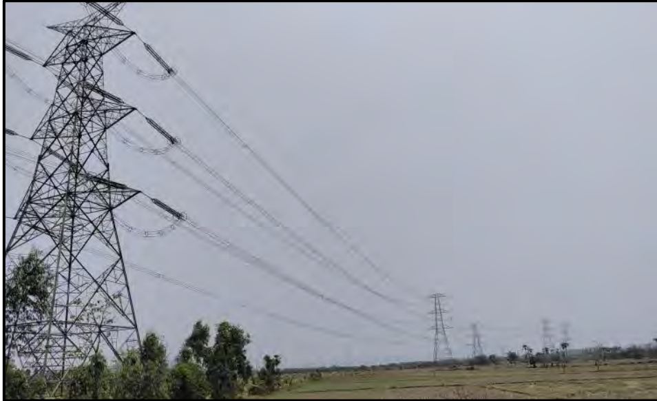
Angle Tower of 765 kV Transmission Line
