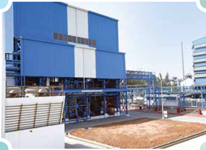
Tarapur Manufacturing Unit II
