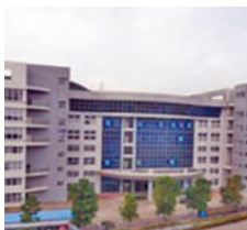
● Igarashi Electric Works (Shenzhen) Ltd, China
