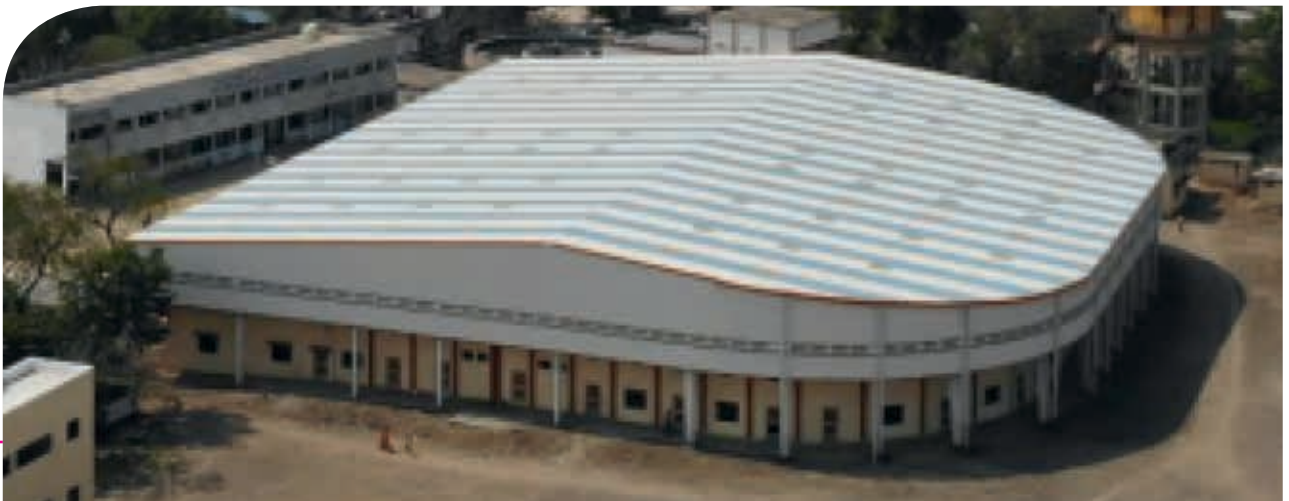
Pre-Engineering Building (PEB)
