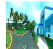
KSB MIL Controls Ltd. Meladoor, Kerala
