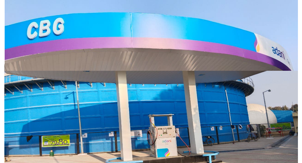
Project Site at Barsana
