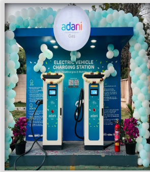
Lucknow Airport, Uttar Pradesh
