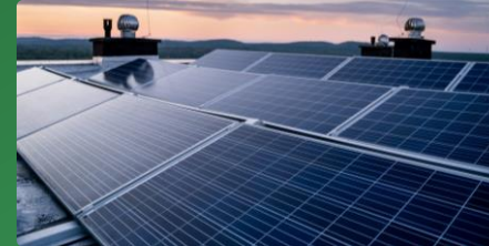
Solar Rooftop Installation
