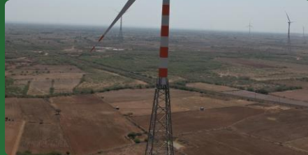
Windmill Lattice Tower
