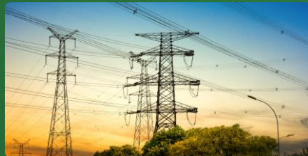
Transmission Line Tower
