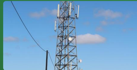
Telecom Tower Structure
