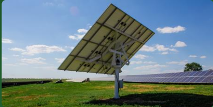
Solar Module Mounting Structure
