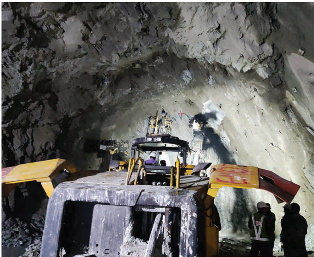
Diversion Tunnel Excavation
