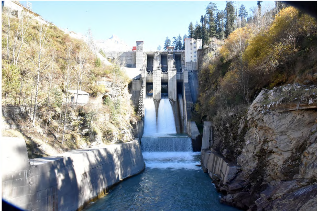
800 MW Parbati-II Project (Himachal Pradesh) – Dam
