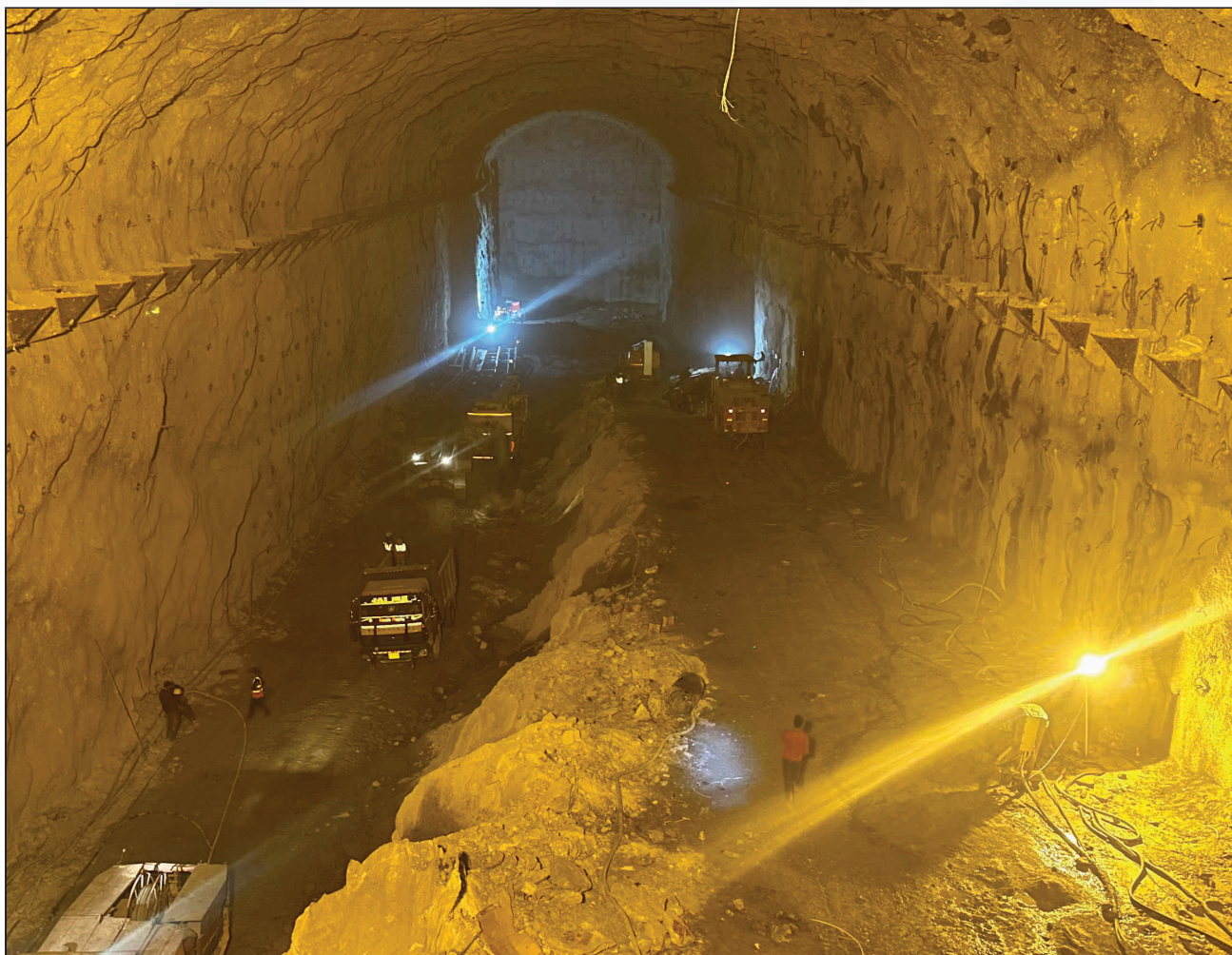
Power House Excavation
