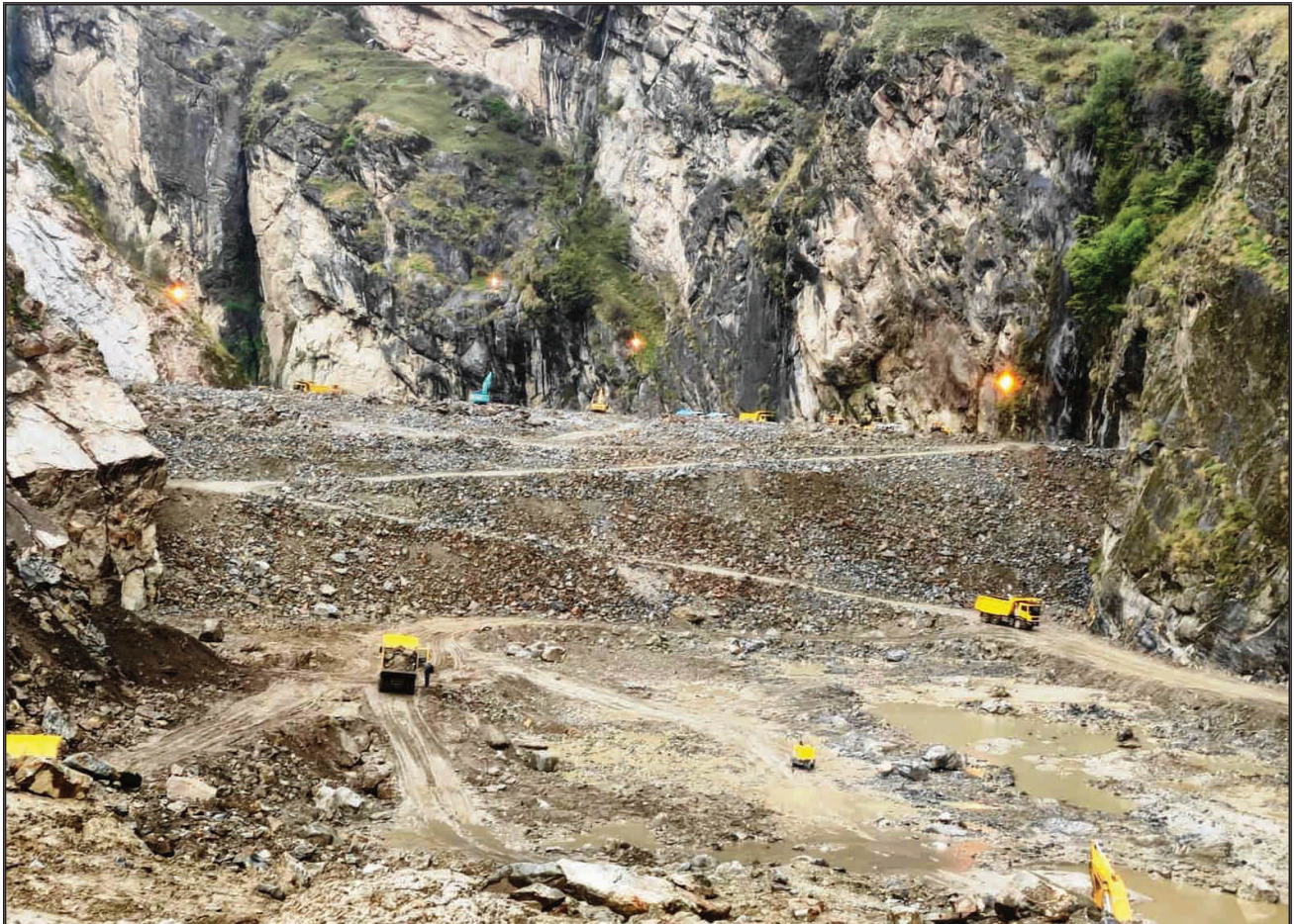
CFRD Dam Filling
