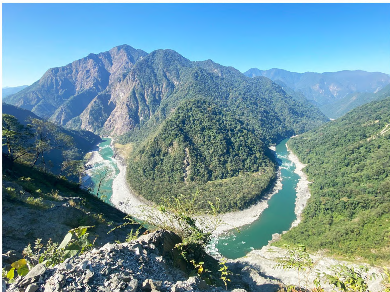
2880 MW Dibang Multipurpose Project Site - Arunachal Pradesh
