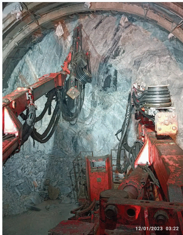
HRT by DBM- In Progress
