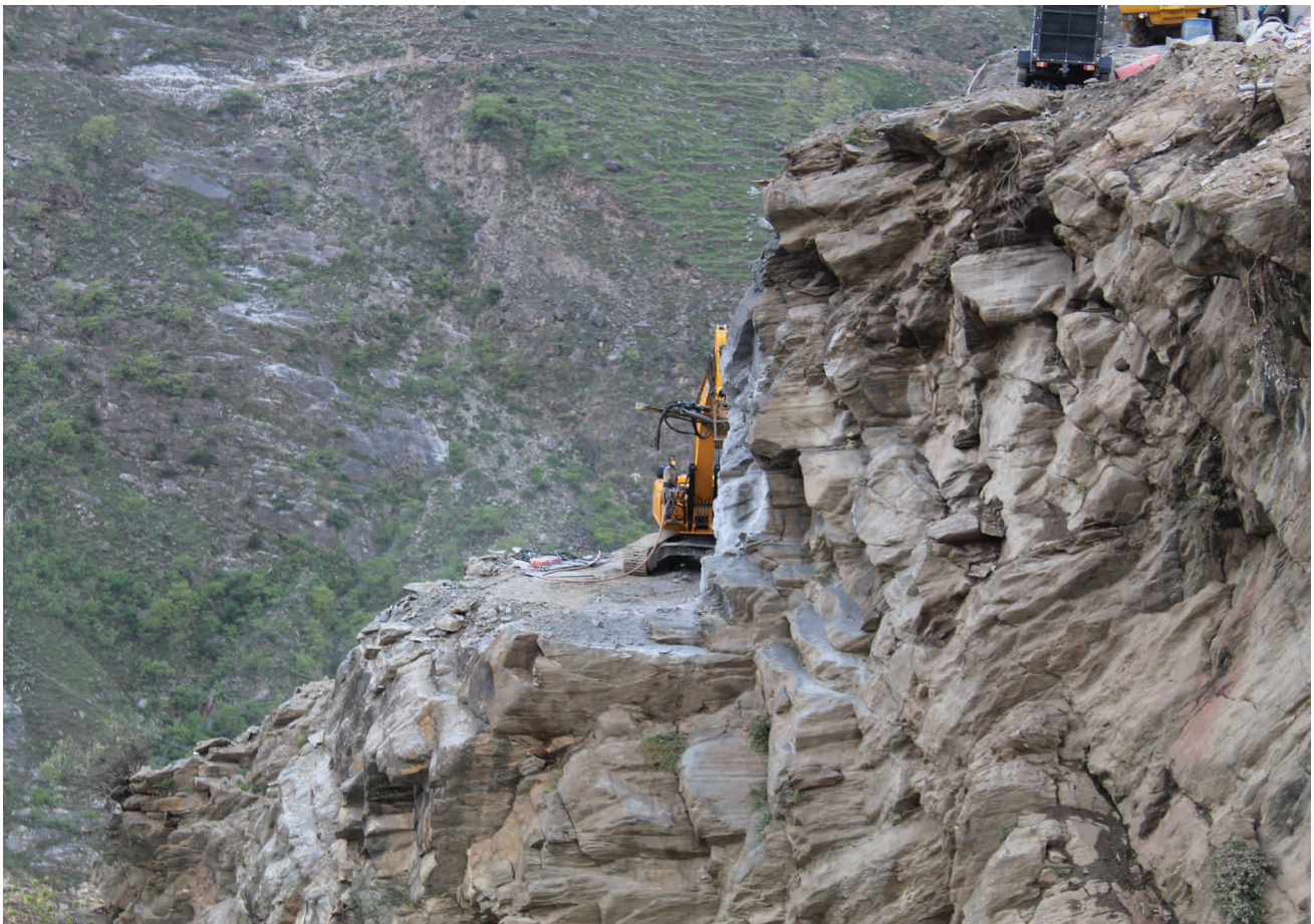
Dam Abutment Stripping
