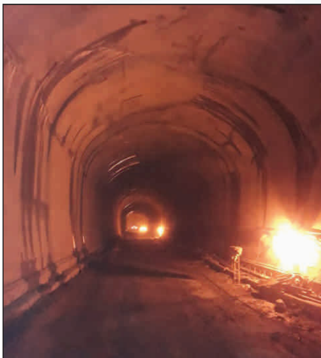
Lining of Access Road Tunnel to Dam site in progress
