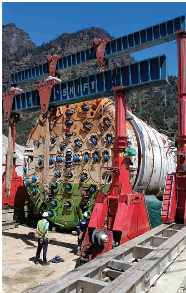
TBM-1 Assembly
