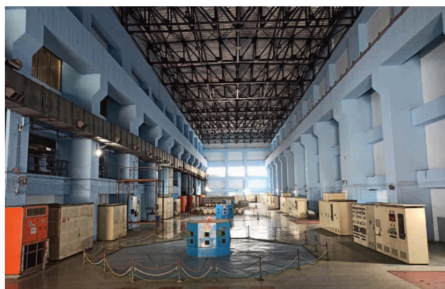
POWER HOUSE: Completed
