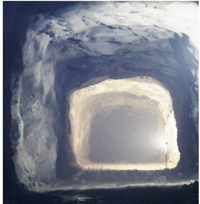
Power House Cavern Excavation
