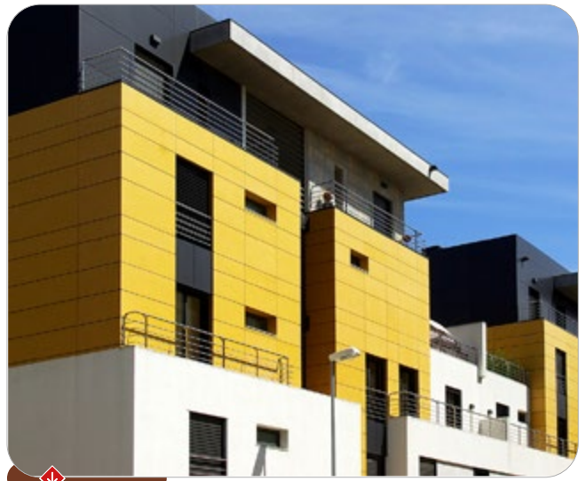
Exterior cladding: fascia
